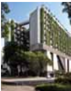
School of the Arts Singapore, 2010 Building Height: 56 meters Stories: 10
