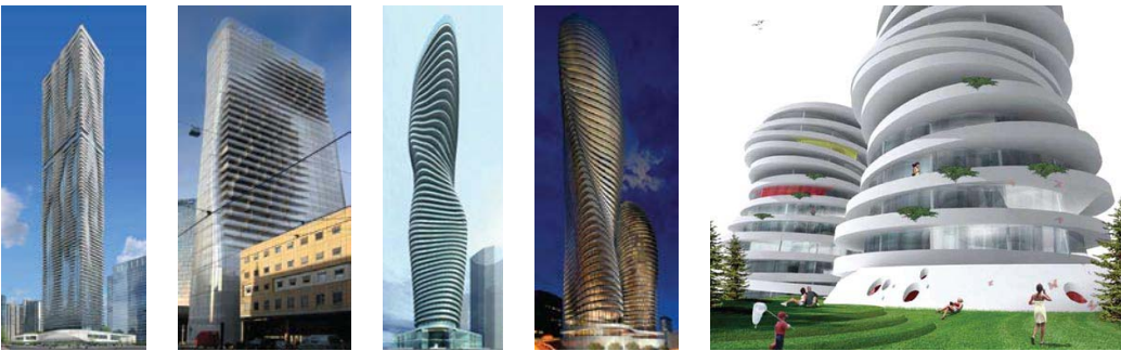
Figures 12a-e. Aqua tower, Chicago, -2009 (© Studio Gang); Tower, Oslo, Norway (© MAD); Absolute World 1, Mississauga, Canada, -2010 (© MAD); Slinky Twins, Paris (© PCA); Nordhavn Residences, Copenhagen (© 3XN)
