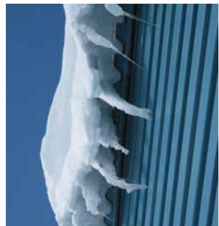
Figure 3. Example of hazardous ice formation on a ledge. © NMI
